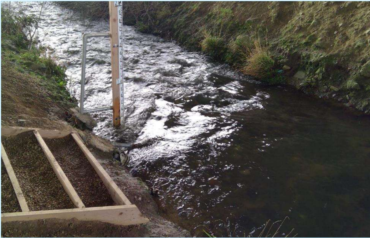
Figure 2-3: Gauge 10048 facing downstream and showing eroded left and right banks.
