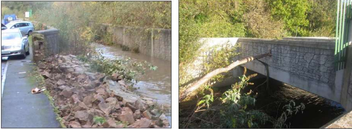
Figure 2-30: Left: Collapsed wall along Commons Road, Right: Tree stuck at upstream face of pedestrian access bridge (Source: Commons Road, Shankill Preliminary Assessment of Flooding Incident 24th October 2011, RPS)
