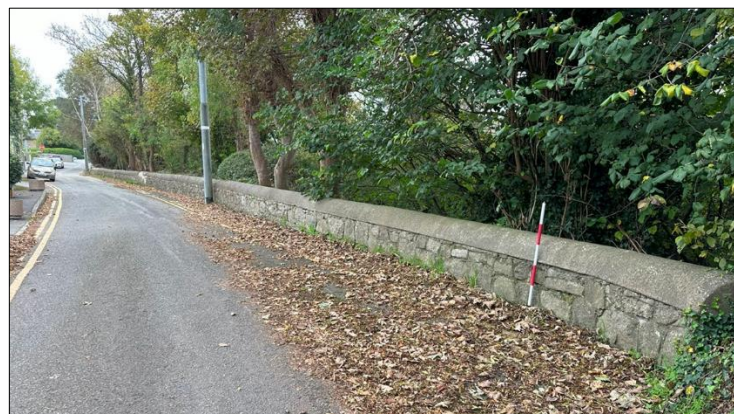
Plate 13 View east along the existing rubbles stone river wall along eastern end
