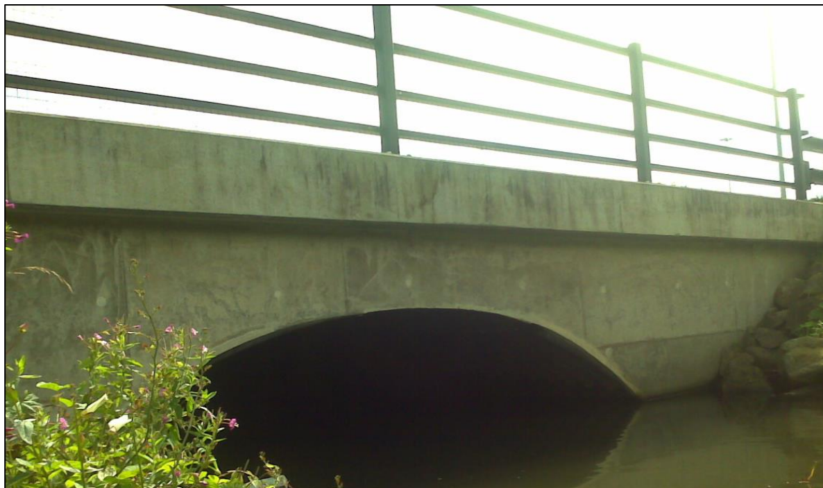
Figure 4.10: Metal railing parapet at Glenamuck Roundabout where flow overtops road
