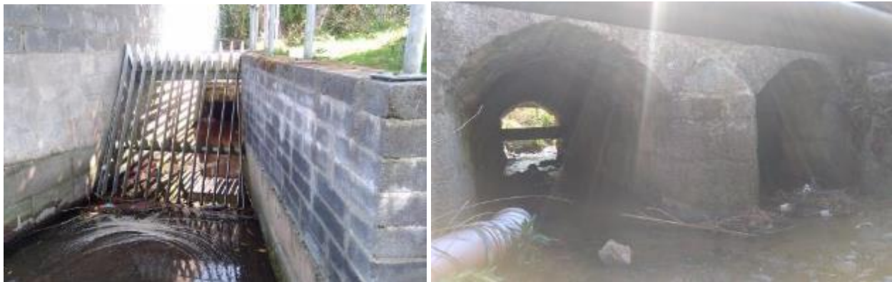
Figure 3.5: Left Inlet of Belarmine culvert, Right – Upstream face of Kilgobbin Road Bridge
