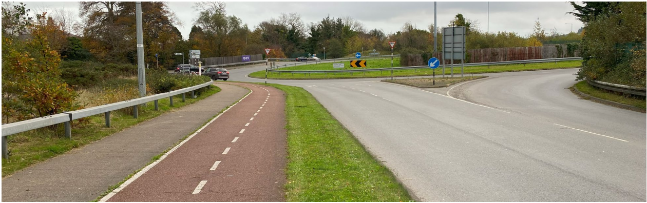
Figure 11.8: Glenamuck Road North (East-West direction)
