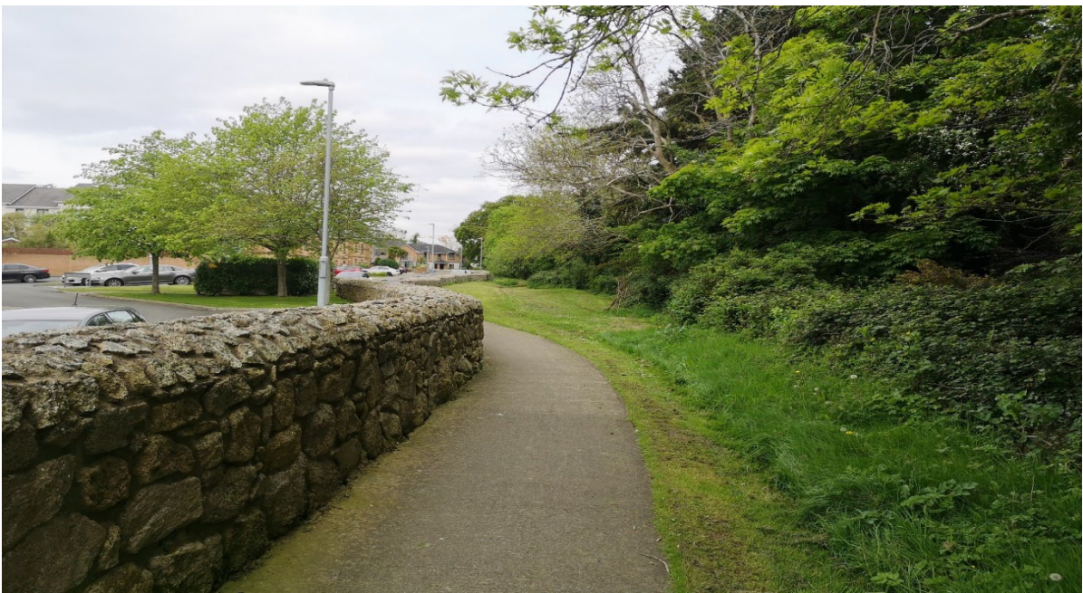
Figure 14.2: Images of Clon Brugh existing stone wall to be upgraded and re-aligned.
