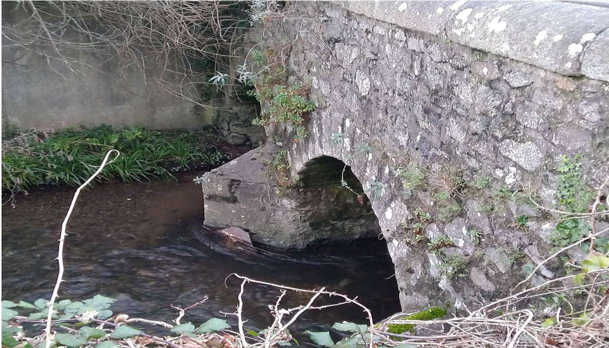
Figure 14-16: Image of bridge on Shanganagh Road
