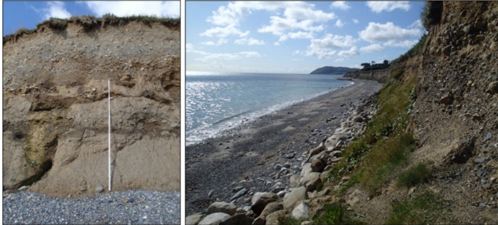
Figure 9.5: Left: An example of layered glacial till; Right: Coastal protection measures ‘rock armour’ boulders
