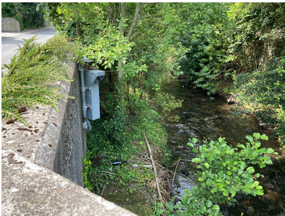
Figure 8.25: The lower section of the Shanganagh River (FW1) is confined by the walls on each bank.
