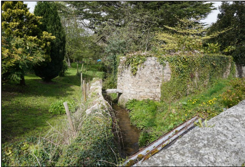
Figure 13.32: Existing view upstream from Kilgobbin Bridge with the curving boundary wall on the right-hand side of the image, the granite slab spanning the river and the low river wall on the left-hand side.
