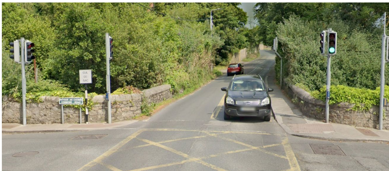
Figure 11.19: Shanganagh Road (Bridge Section)
