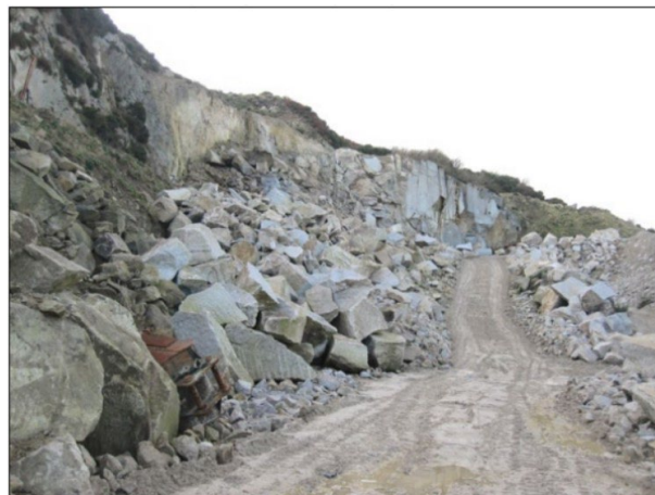
Figure 9.4: Murphystone Quarry as seen from the entrance 29
