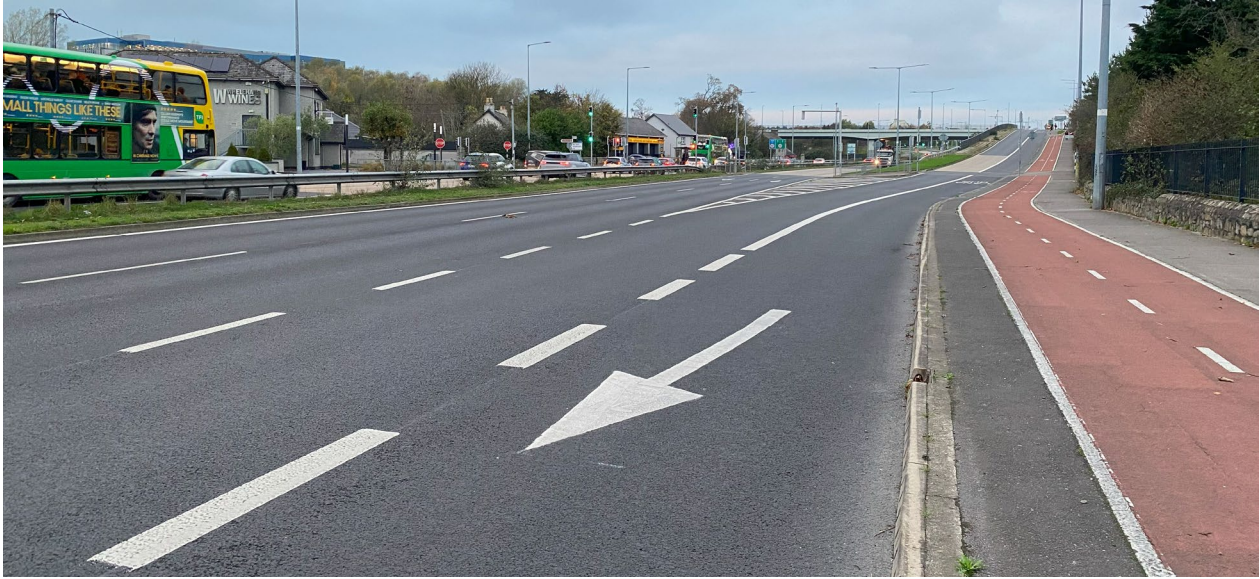
Figure 11.13: N11 Southeast Bound at the Location of N11 Crossing Site
