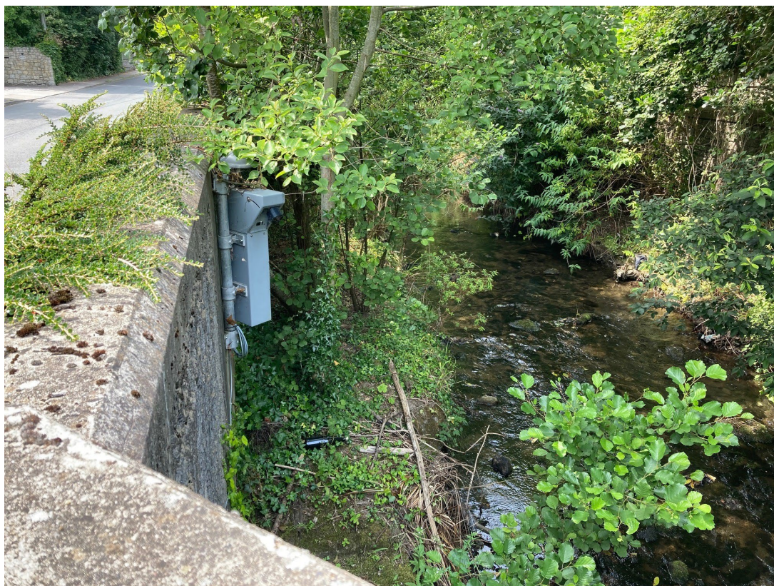
Figure 3-20: The lower section of the Shanganagh River (FW1) is confined by the walls on each bank.
