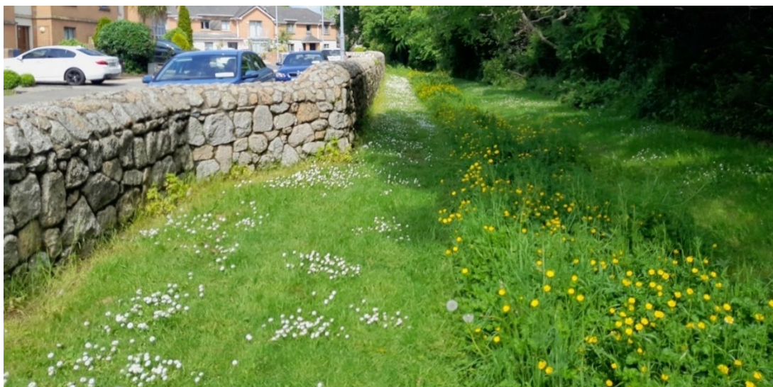
Figure 3-3: The ditch running through the Clonbrugh stretch of the scheme, with the distinct floral diversity visible in contrast to the amenity grassland on either side.
