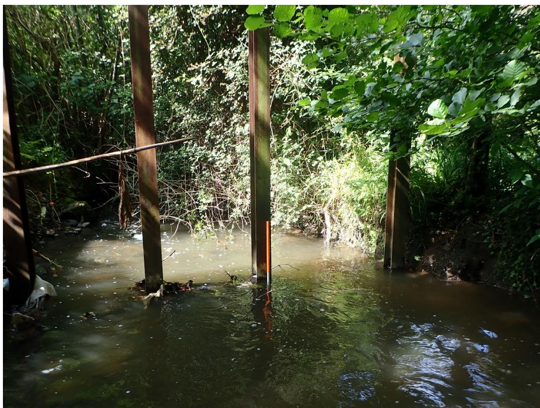
Plate 10: Debris trap inserted into the Shanganagh River in the recent past.
