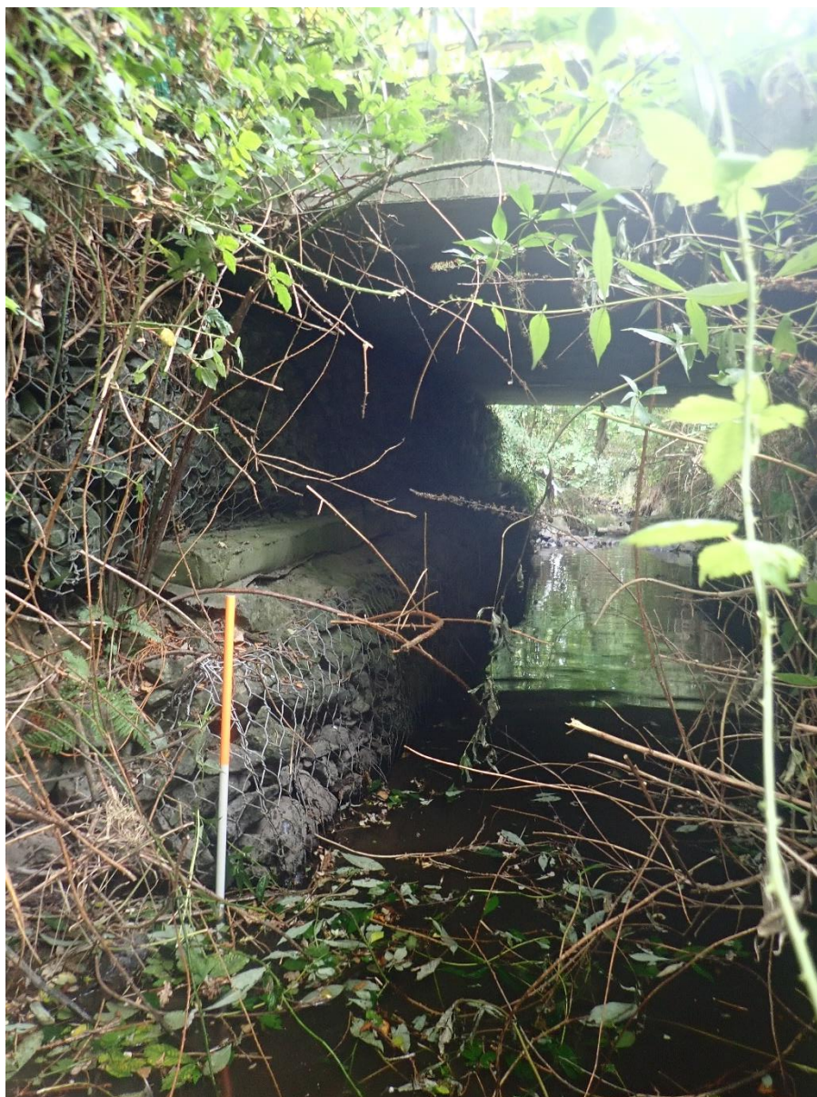
Plate 16: Modern bridge replacing U115, Loughlinstown River North.
