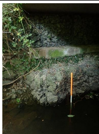
U115, site of, showing base of modern bridge, right bank
