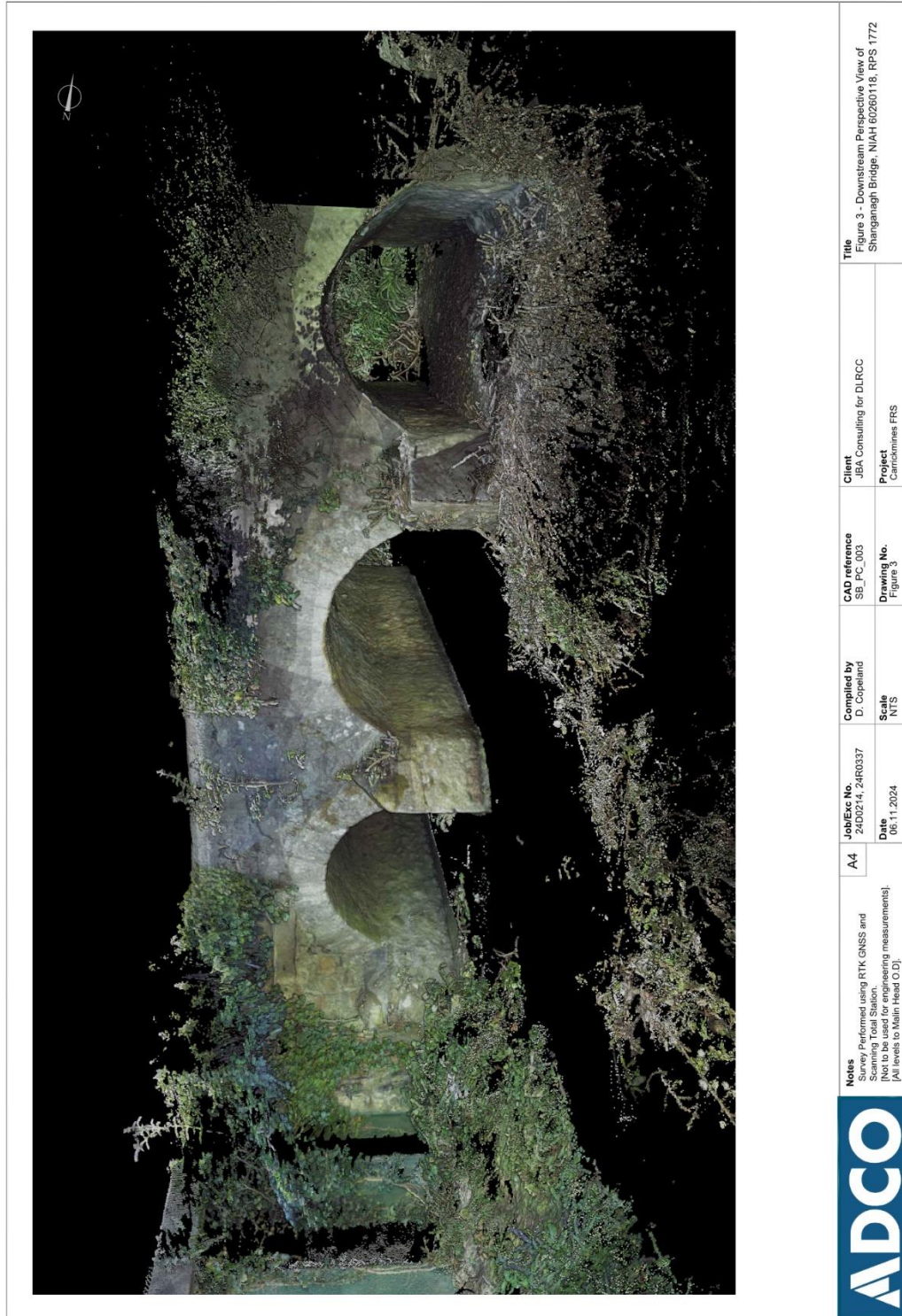
Figure 3: Point Cloud image derived from laser scan survey of Shanganagh Bridge. View looking upstream towards bridge.
