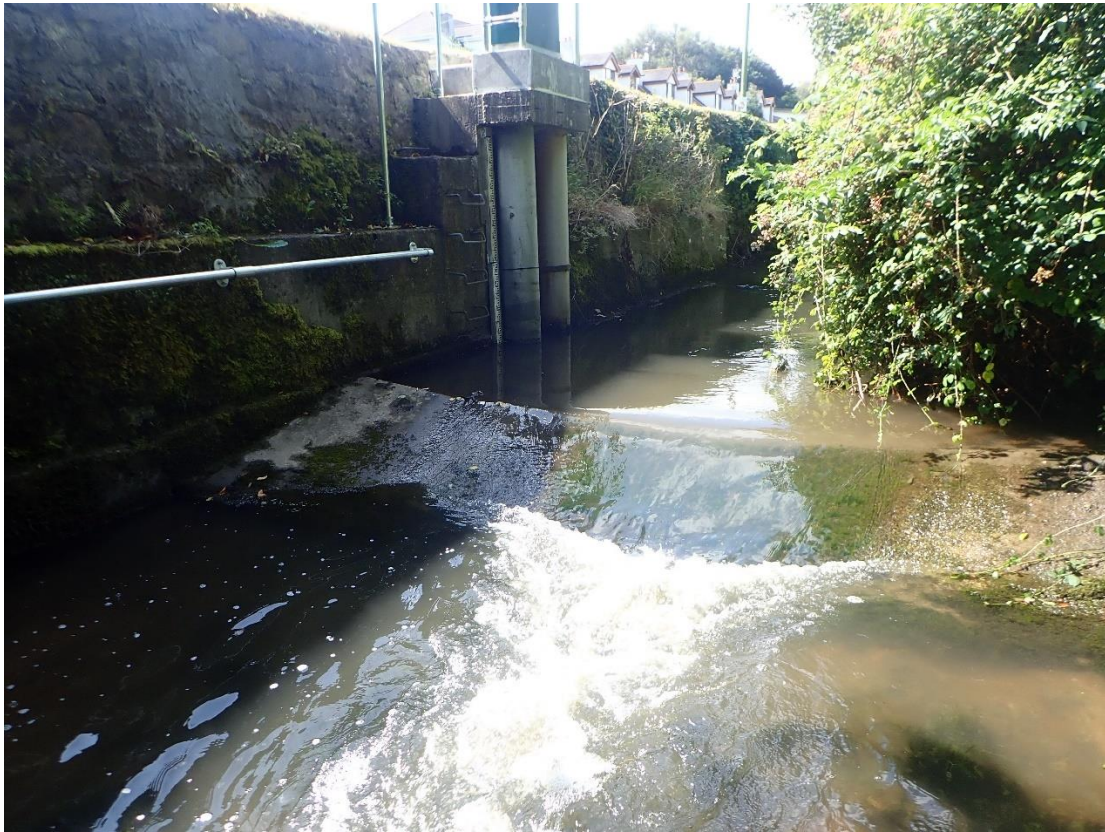
Plate 7: View of concrete weir and flood gauge at upstream limit of UAIA area.
