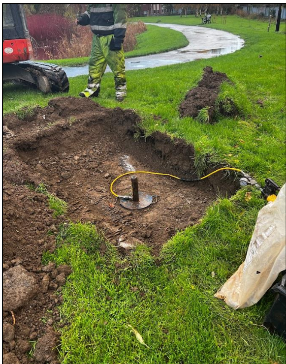
Plate 4: Plate test at Belarmine.
