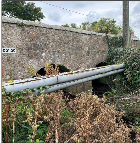
Upstream facing façade of the bridge.
