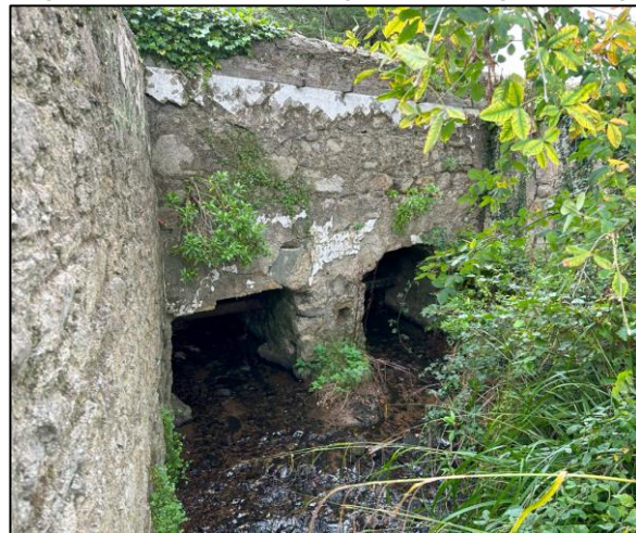
View of the downstream façade of the bridge
