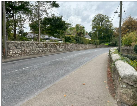
Kilgobbin road view looking south along the bridge
