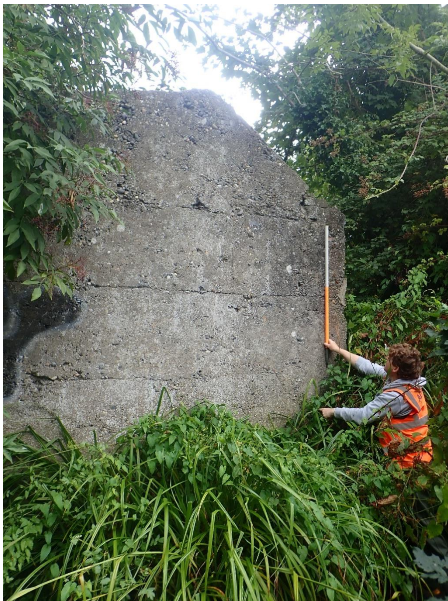
Plate 19: View looking north at rear wall of outhouse that occupies one of the now-commercial premises on the old Bray Road. The poured concrete-and-pebble temper mix is typical of early 20th-century dwellings in the wider area.
