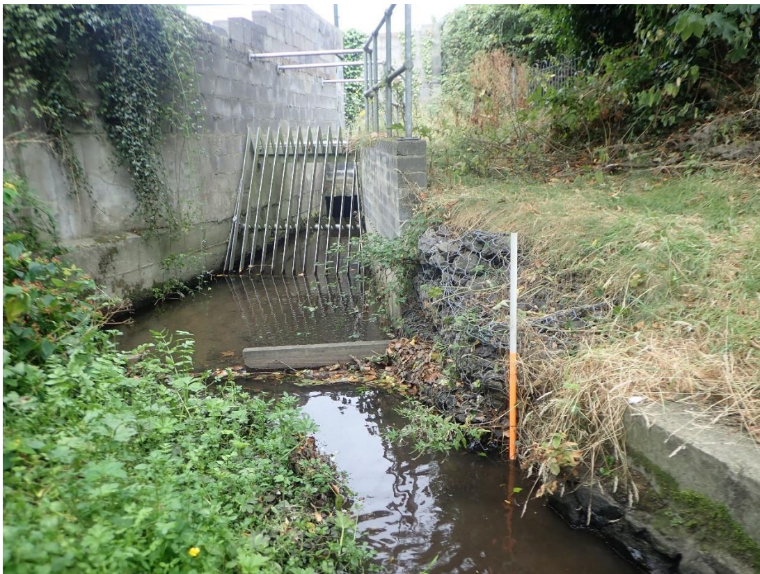
Plate 28: View of Kilgobbin Stream in Belarmine Park where it is culverted.
