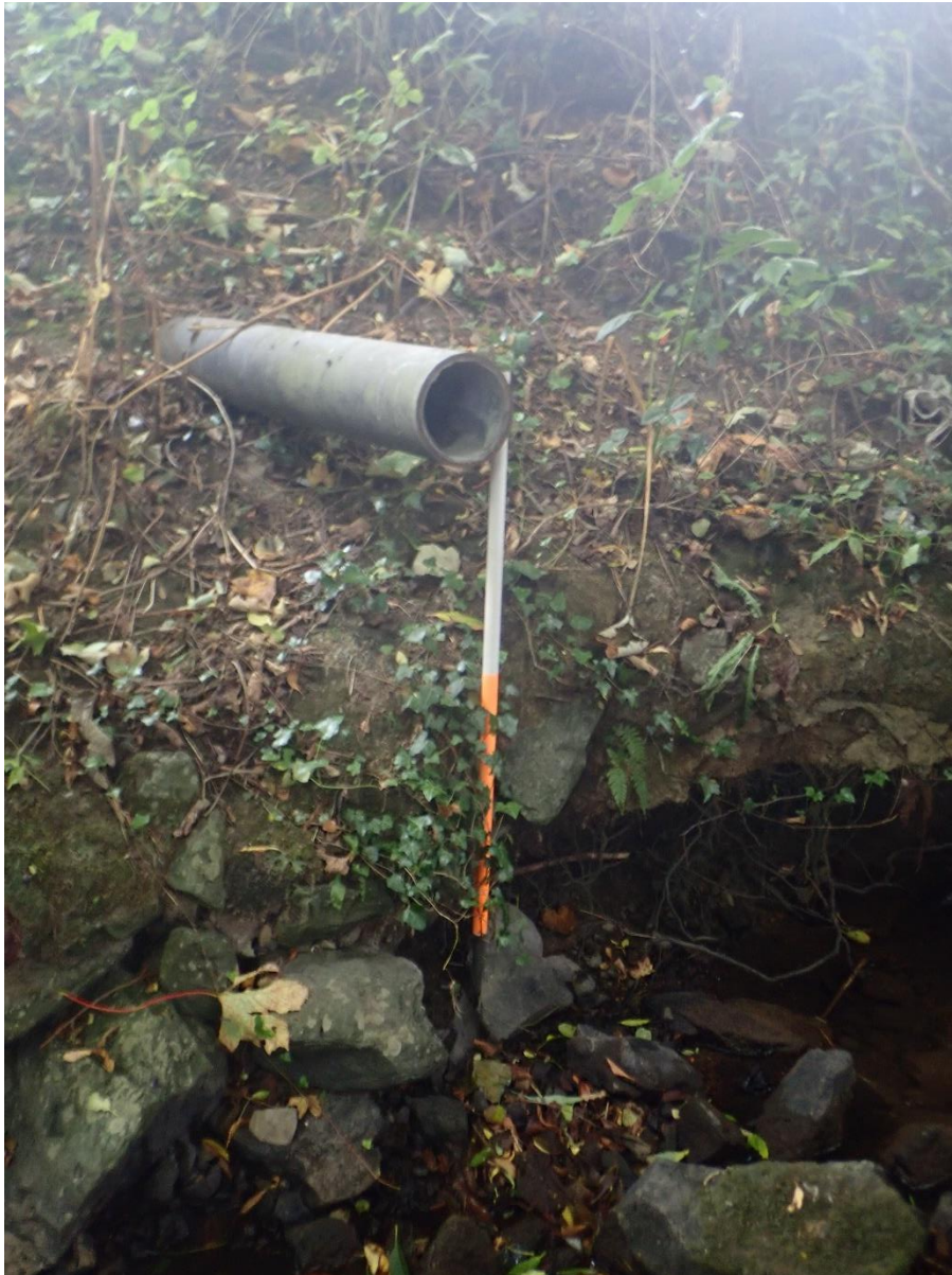
Plate 15: Example of pipe entering Loughlinstown River North from the left bank.
